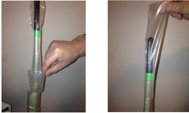
Figure 15. Removing the outer cover.
